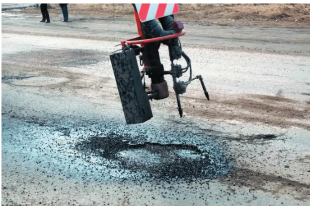
Figure 1. Injection of injectable material
