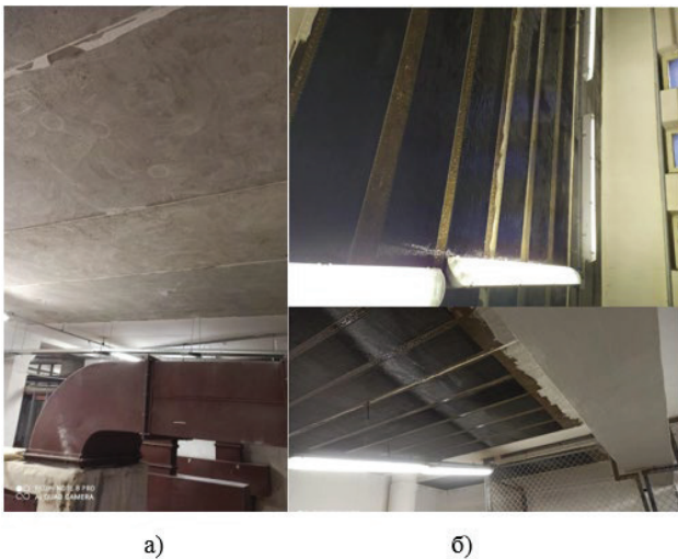
Figure 11. Structural elements of the building of the Government House of the Russian Federation: a) before reinforcement; b) after reinforcement with composite ERS
