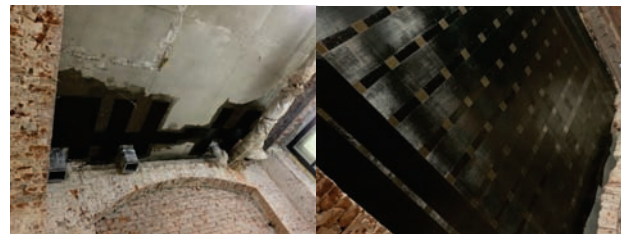
Figure 10. The appearance of the reinforced structures of the History Museum building
