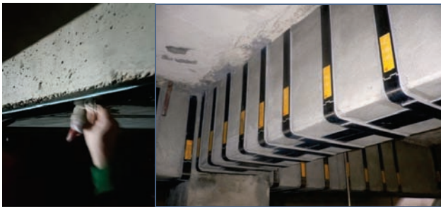
Figure 8. Installation of Fibarm Laminate lamellas
