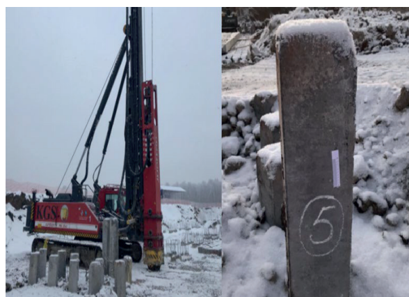
Figure 3. a) Junttan PM-25HD piling rig in Nur-Sultan city, b) test pile
