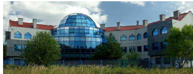
Figure 1. General view of the CUS building in Psary.
