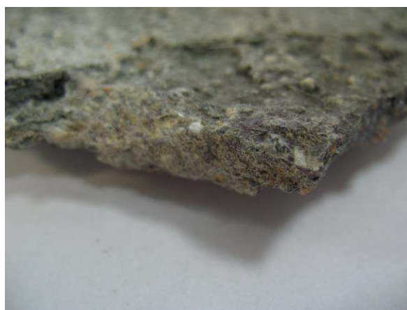
Figure 2. One of the real specimens of repair composition with sulfatized layer on the inner side.
