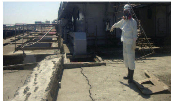
Figure 13. Formation of the main crack in the base plate (Fukushima I, 2011)
