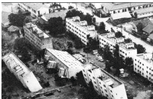
Figure 12. Failure of buildings caused by soil liquefaction (Niigata, Japan, 1964) by FEMA
