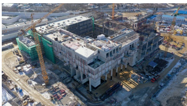
b) Construction stage
