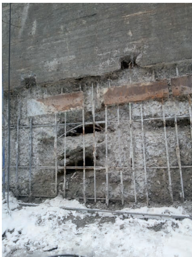
Figure 4. View of a wall with sloping cracks extending to the face, with voids, exposed reinforcement and water leaks (before overhaul)
