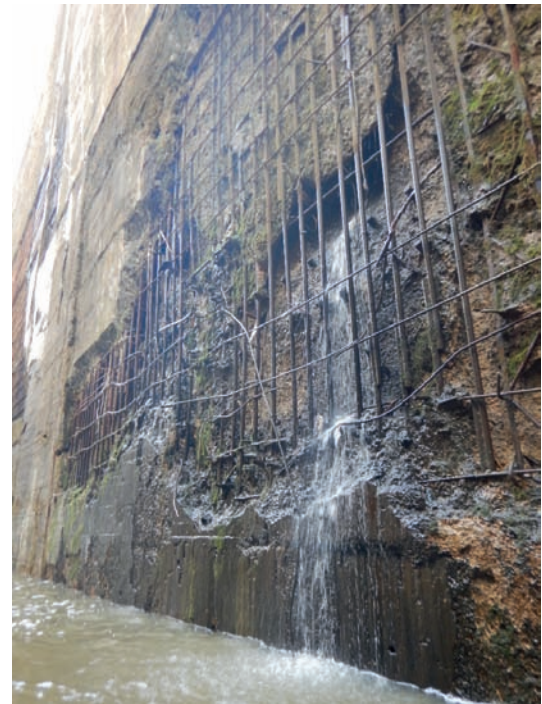
Figure 2. View of the right wall of section No.1 with a sloping crack extending to the face, with voids, exposed reinforcement and water leaks (before overhaul)
