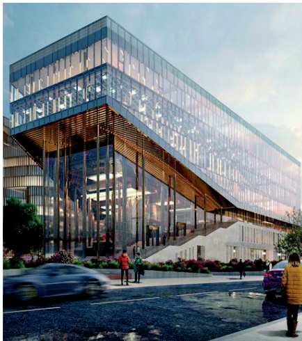
Figure 2. Investigated Building with CSGF
