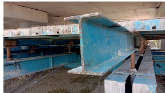
Figure 6. WF 150.75.5.7 (After installation)
