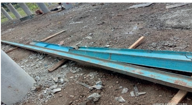
Figure 5. WF 150.75.5.7 (before installation)
