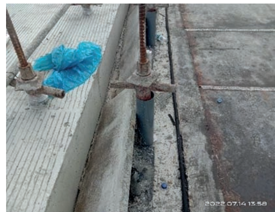
Figure 12. PT Bar Washing at Pile Head
