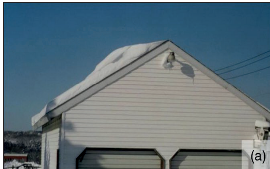
a) snow distribution on a gable roof (from [9])
