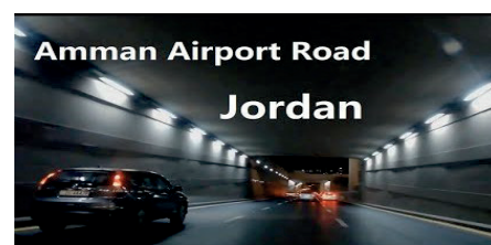
Figure 2. Tunnel Project in Amman (Researcher)
