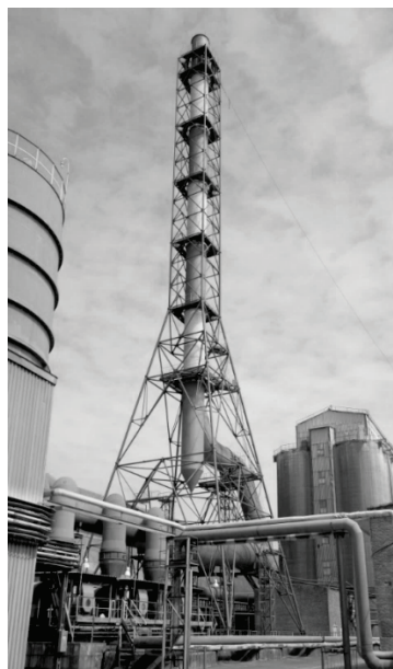
(a) A chimney in a cage
