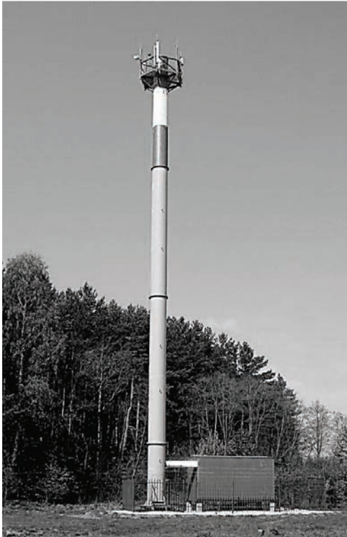
Figure 3. The pole with a height of 35 m
