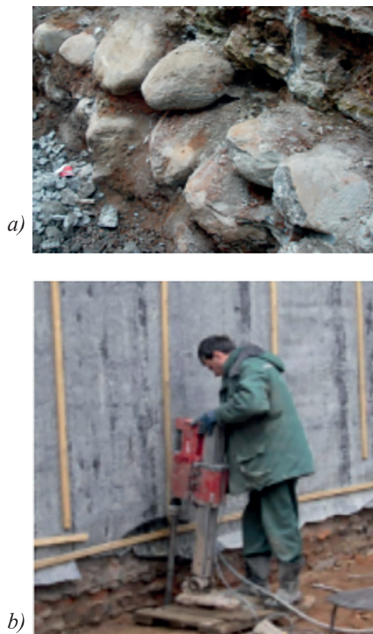
Figure 4. Underpinning of foundations and ground bed of building in Stremyannaya Street (a and b)
