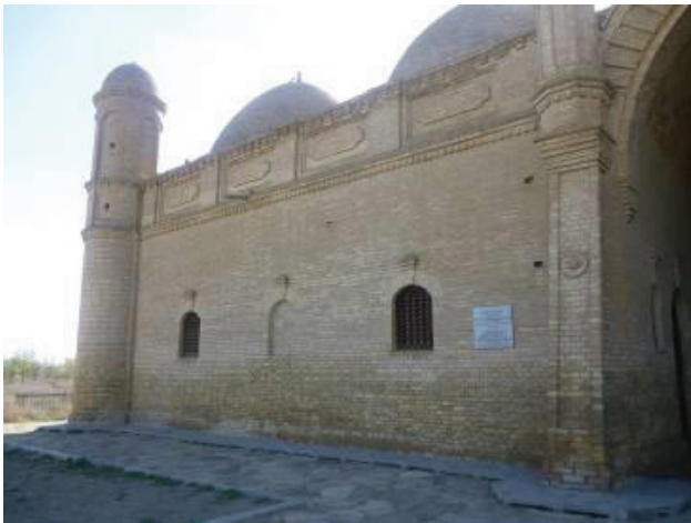
Figure 7. Moistening of the Lower Part of a Northeast Facade of the Mausoleum Arystan-Bab.
