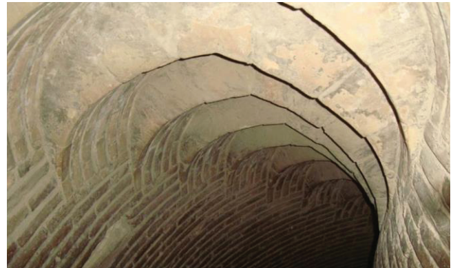
Figure 9. The Arch of the Spiral Staircase of the Minaret Kalon.
