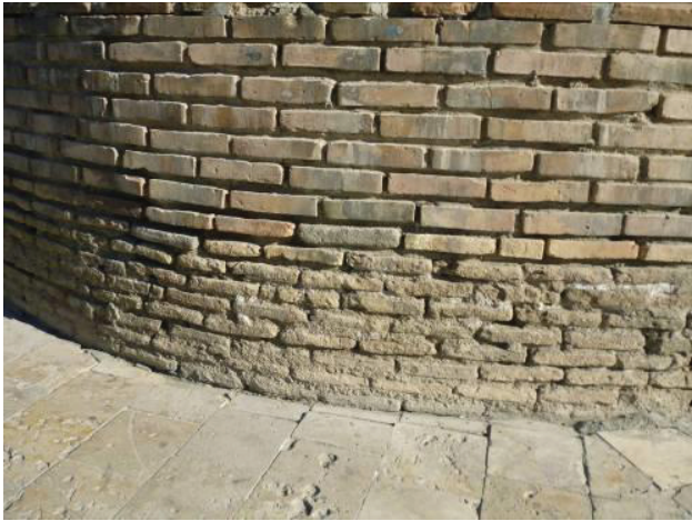
Figure 10. Aeration of Solution in Bricklaying Seams of Mosque Kalon.
