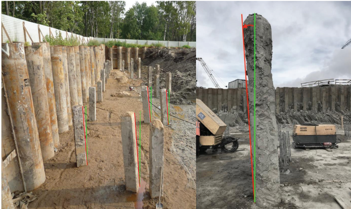
Figure 1. Horizontal displacements of driven and bored piles.
