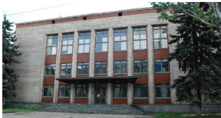
Figure 2. Building before reconstruction.
