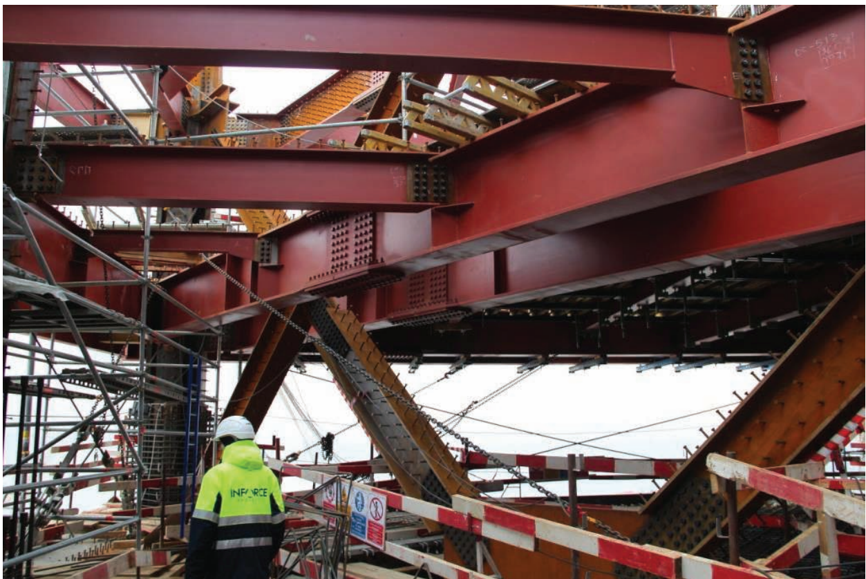
Figure 8. Building of metal structures of outrigger level.
