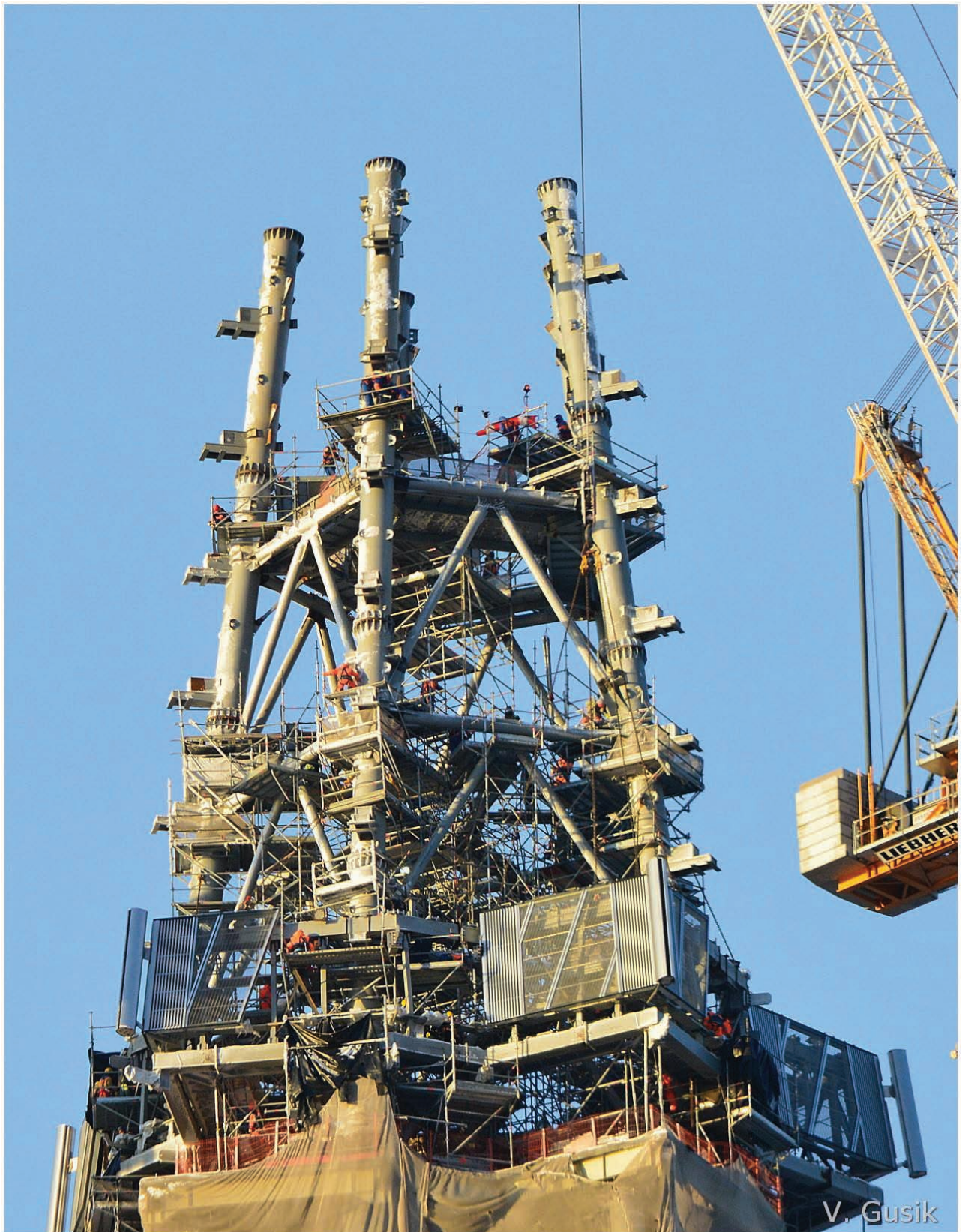
Figure 10. Mounting the spire.
