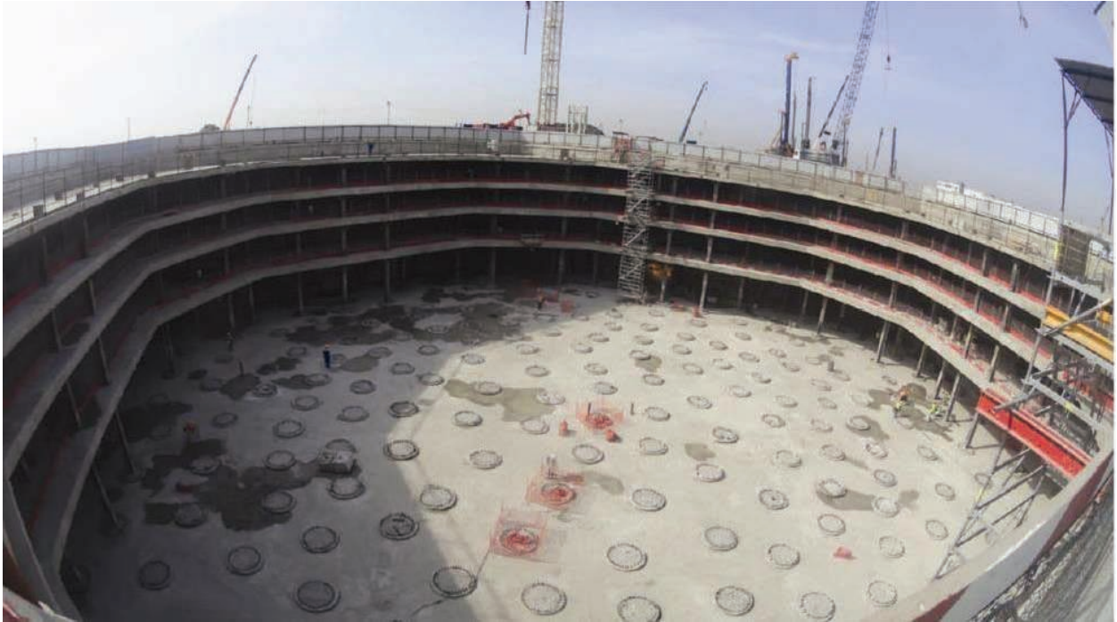
Figure 4. General view of the pit after excavation until design mark and preparation for concreting.
