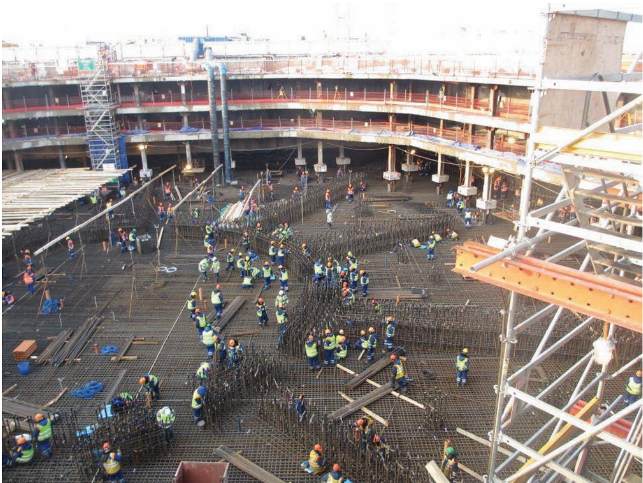
Figure 5. Reinforcement of the bottom plate of the box foundation.
