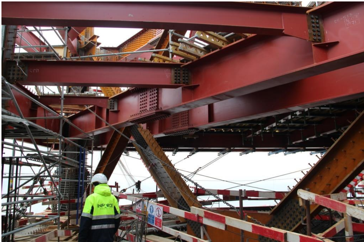
Figure 8. Building of metal structures of outrigger level.
